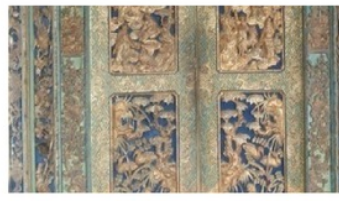
Figure 3. Detail of ornaments on door in Maskerdam building
