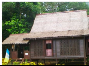
The traditional Malay house architecture with three ridges and carved patterns of even arabesque elements on the wooden walls
