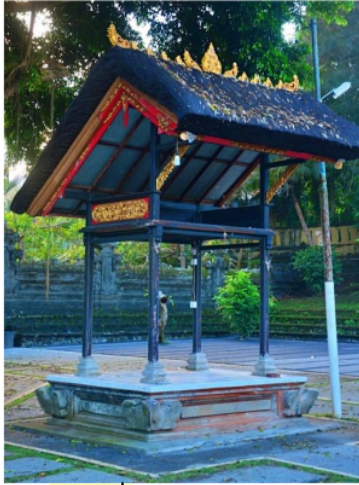
Fig. 6: Original architecture of Bale Patokan. Source: Author, 2023.
